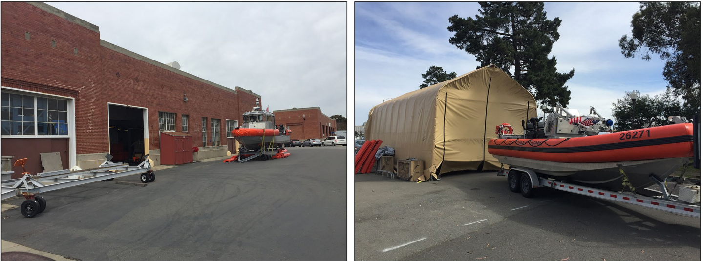
Figure 1: Coast Guard Maintenance Facilities Requiring Refurbishment because They Cannot Accommodate Newer, Taller Boats
